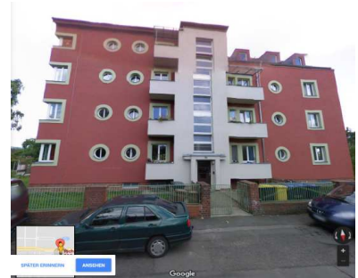
Pilot Project Tenant's electricity in Leipzig's "Südvorstadt"
